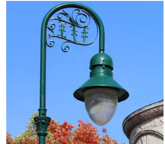
An example from Indiana University of hooded street lighting featuring ornamental elements with a frosted globe to prevent glare.
