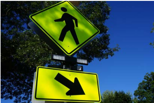
An example of a Rectangular Rapid Flashing Beacon (RRFB) sign.
