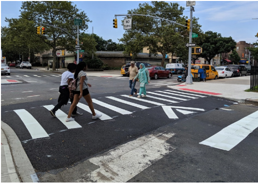
An example of a raised crosswalk in Brooklyn. NYCDOT Street Design Manual.
