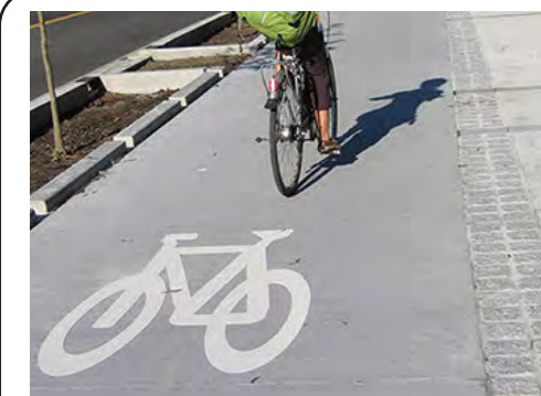
CONCRETE RAISED BIKE LANE
