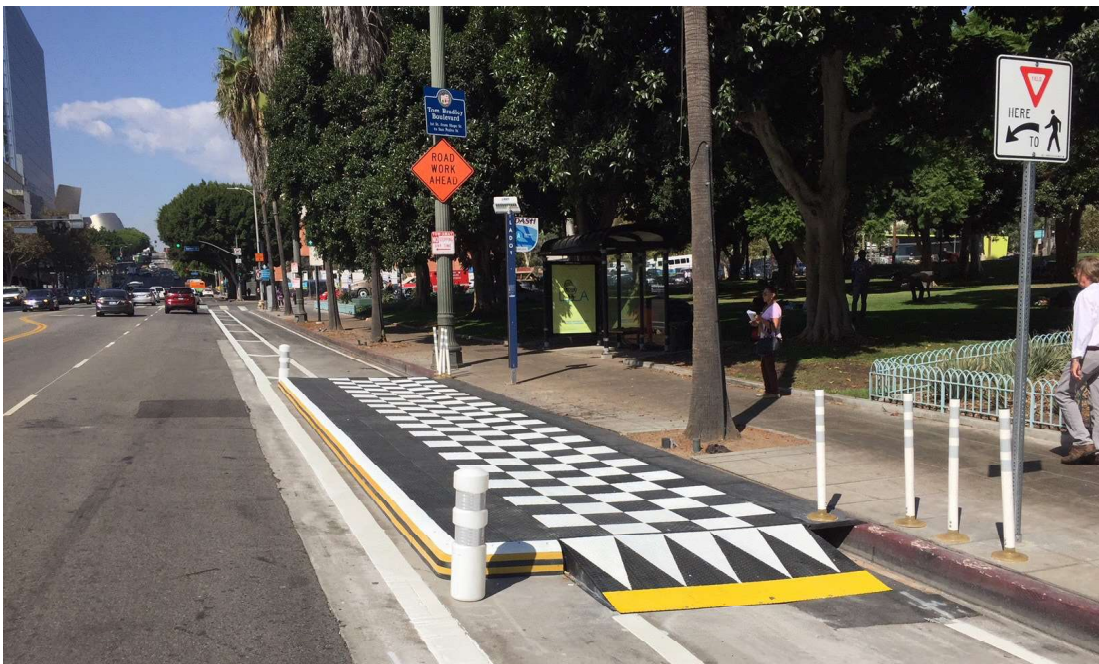
Example of a flexible bus bulb platform with a bicycle lane traversing through. Bicycles must yield to pedestrians. Ramps help slow down bicycles as they approach the bus bulb.
